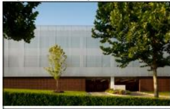
Utilising metal mesh as a facade screening component
